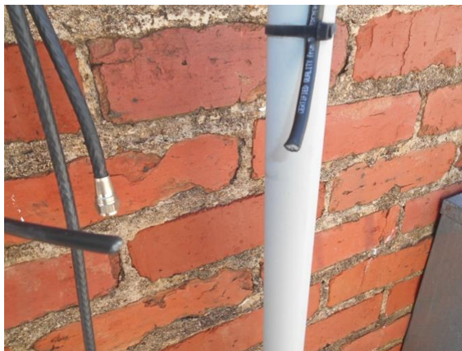
Cut Antenna Coax On 146.85 Repeater
